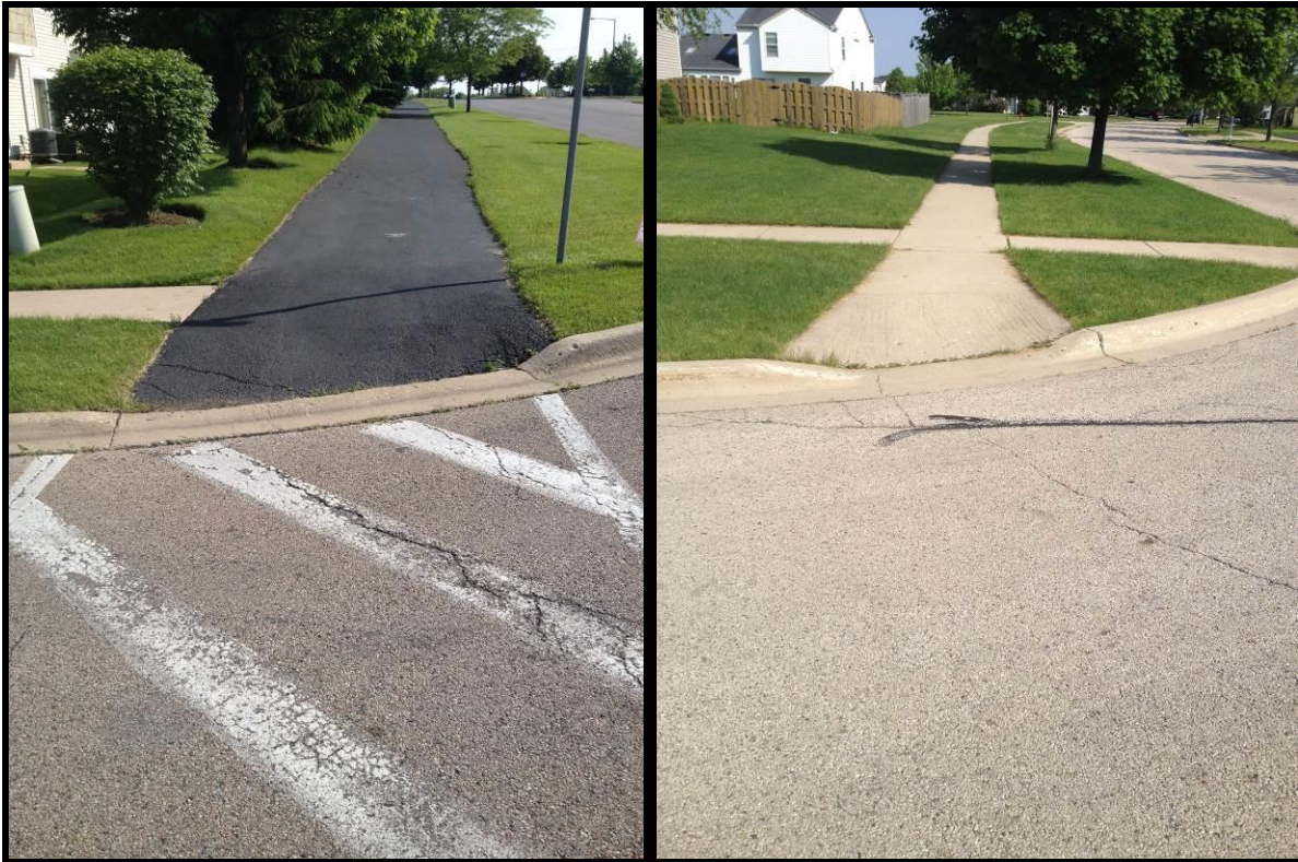
The above curb ramps do not have proper detectable warnings and are “non-compliant” with current ADA Standards. They will be replaced with prefabricated truncated dome panels as part of the Village annual CIP program.
