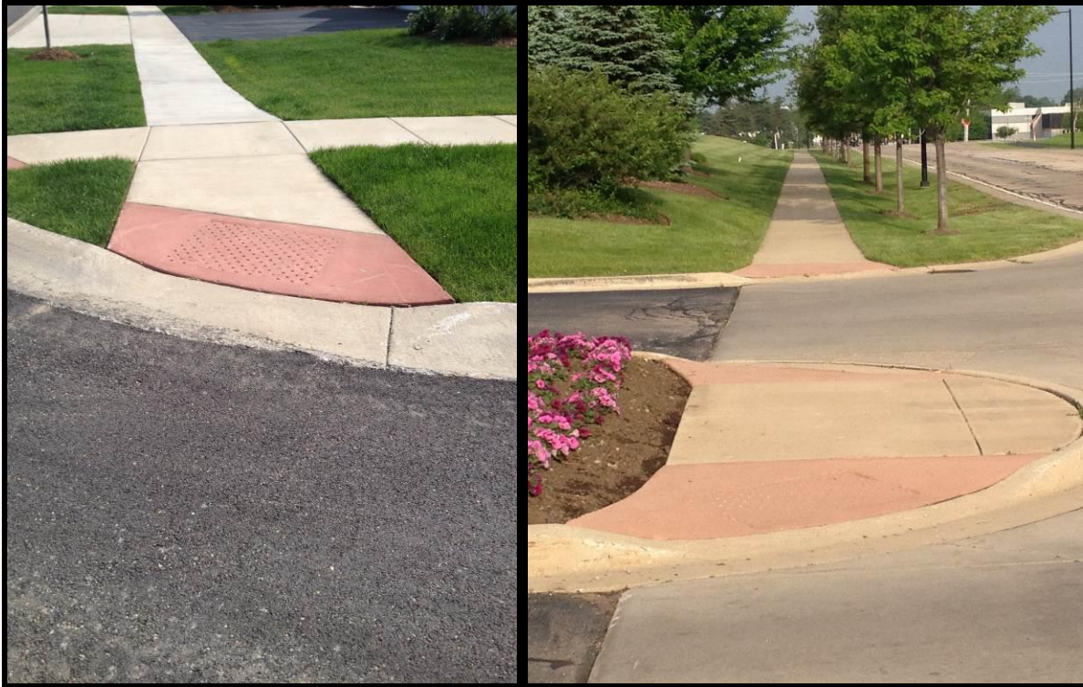
The above detectable warnings are stamped concrete type. They make up the majority of the “ potentially compliant ” transitions in the Village and will be replaced with prefabricated truncated dome panels as part of the Village annual CIP program.
